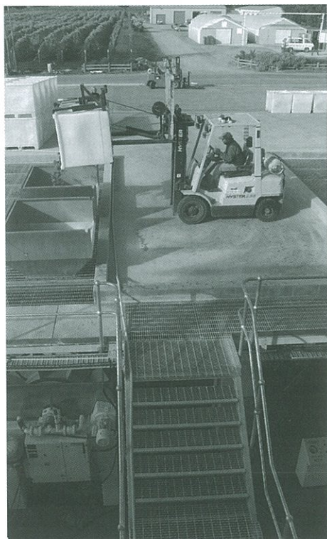
Cloudy Bay's new underground press facility.
